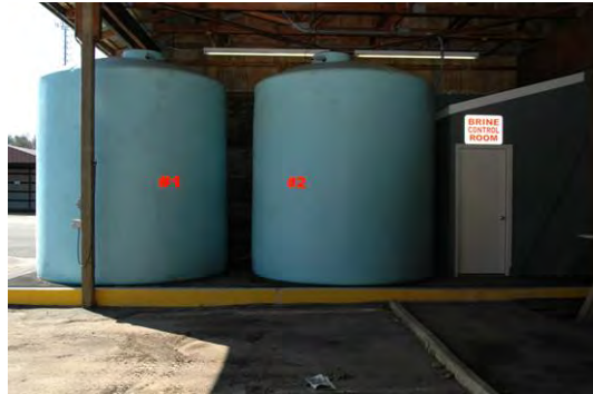
Figure 28. Proper Brine Storage
